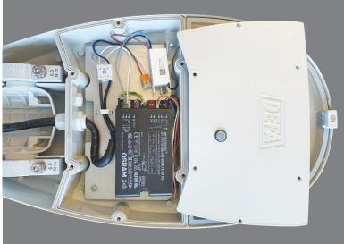
Connect according to wiring diagram and fix photocell to one screw.
